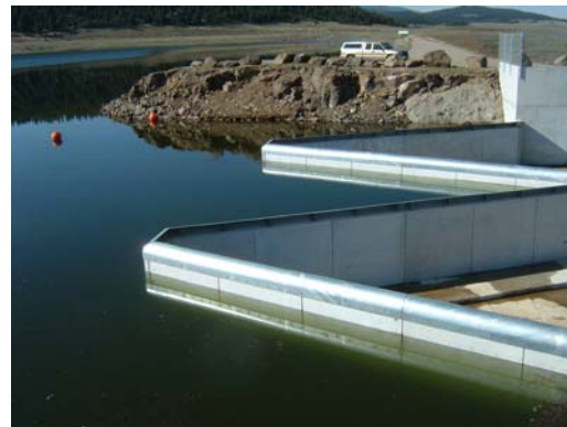
North Fork Smith River Dam (after rehabilitation)
