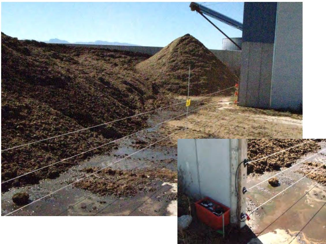
Figure 2. Design and installation of a portable 12v-converted to AC powered electric fence system to deter grizzly bear access into the Pondera Colony livestock carcass compost facility, 9/20/2013.
