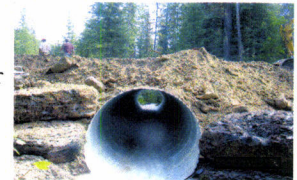
Culvert installed to prevent sediment from entering the
